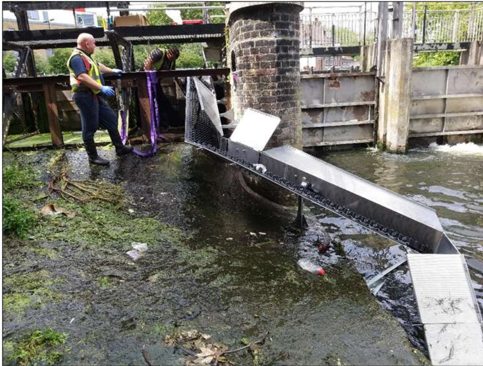
Figure 10. The gravity eel pass at Lea-Lea Bridge under construction in July 2020
